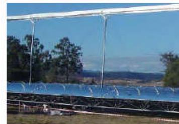
Figure 2.2-4. Linear Fresnel System
